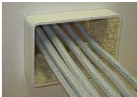
Apply NF-23 so that none of the cables is touching the coaming.
